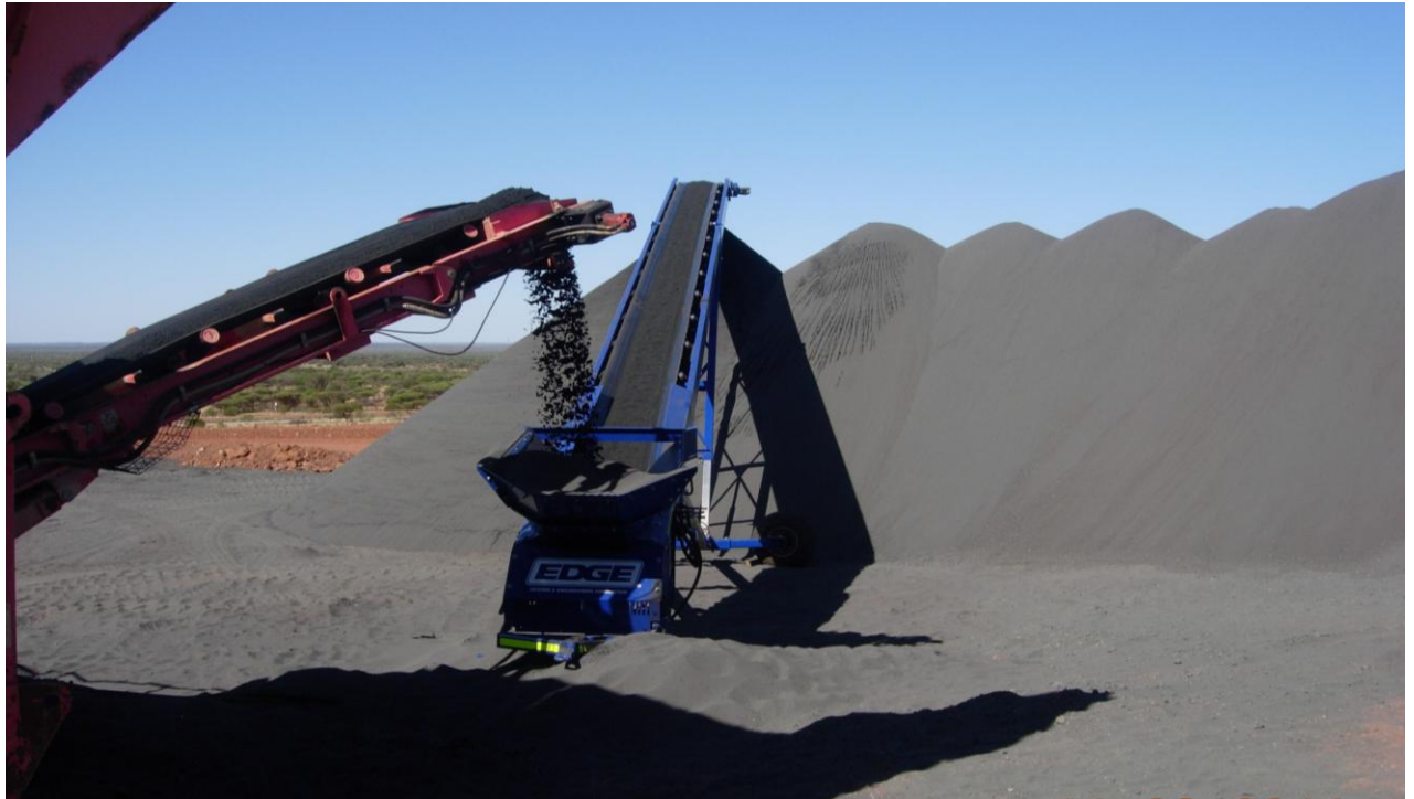
Calcined iron fines undergoing screening and stockpiling
