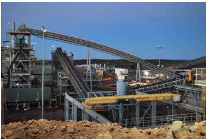
Windimurra Vanadium Project © Atlantic Ltd.
